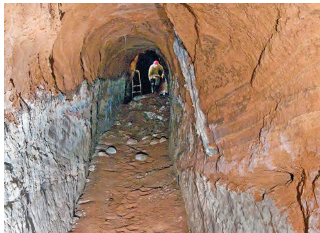
View from the junction to the waterwheel passage, along the main water channel to the access point, where the man is standing. A lot of the debris in the channels (and the canal tunnel) is due to spalling of the sandstone roof, mixed with silt. Again, note the historic water level marks
